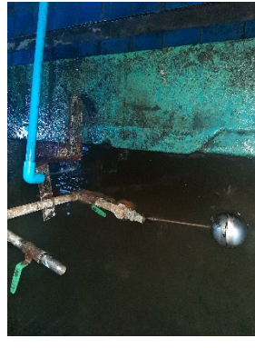
Level is high float not make up
