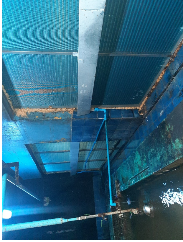
Level is high float not make up
