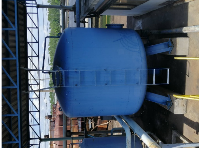
Sand filter tank
