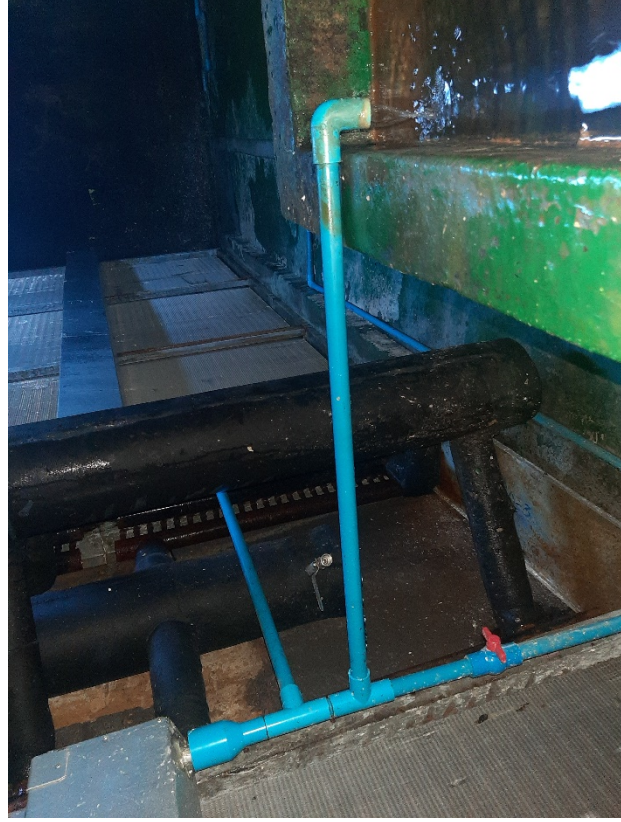
Tray , PVC pipe connect fill to pit
